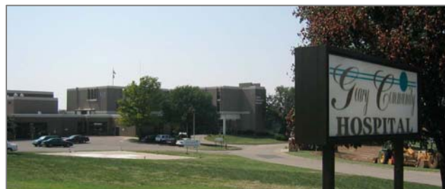
Tractors are at work on expansions to the hospital.
